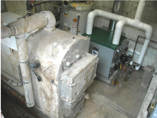
Figure 4. Existing low-pressure steam boiler (left) New low-pressure steam boiler (Right)
